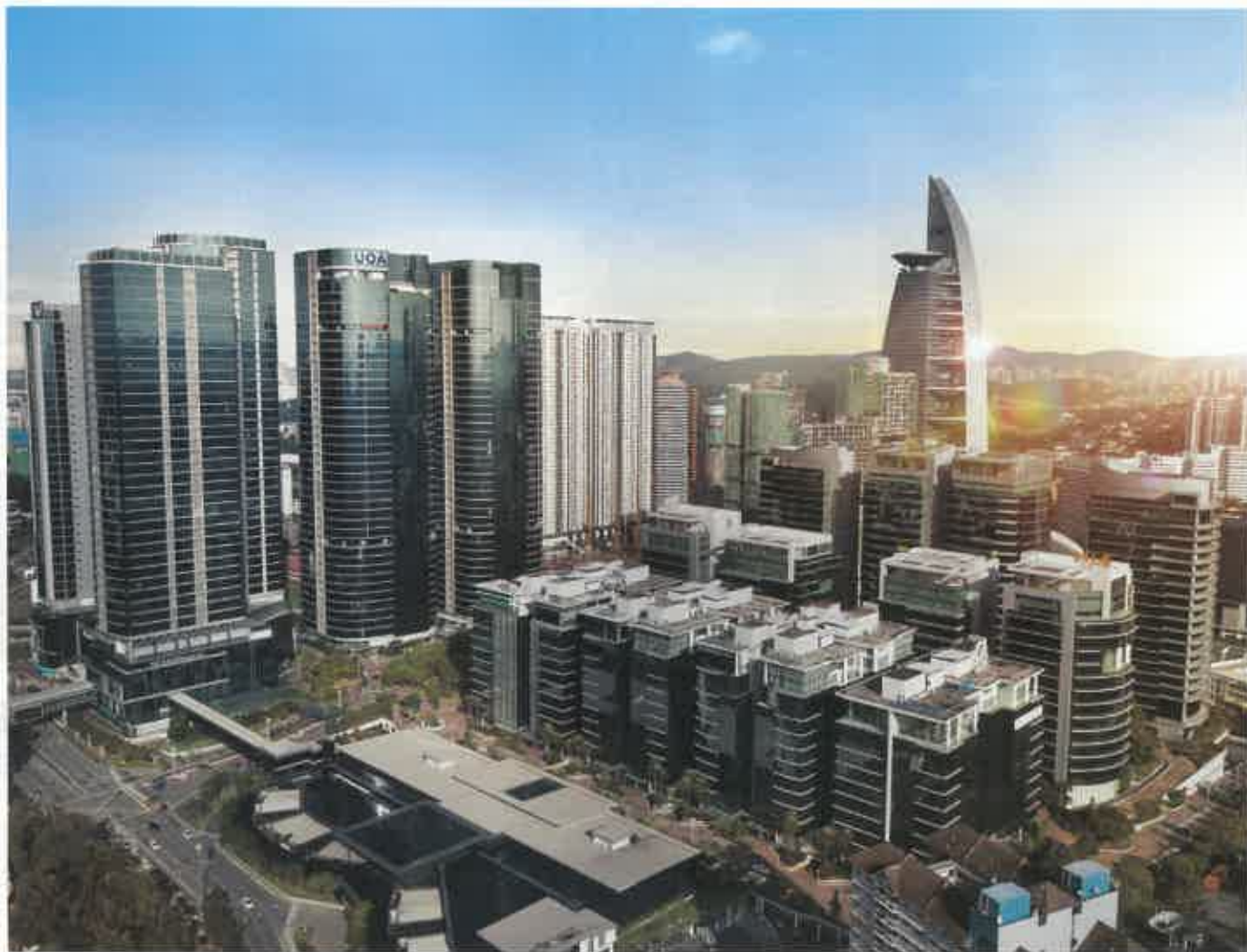
An aerial view of Bangsar South
