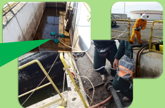
The SMART skimmer intervention has eliminated the source of pollutant and reduced the cost of dewatering.
