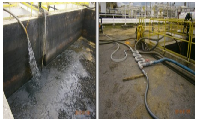
The conventional removal activity is usually took 30 minutes/session that involved three operators.
