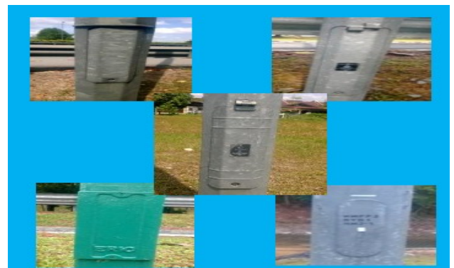
Example of maintenance service doors.
